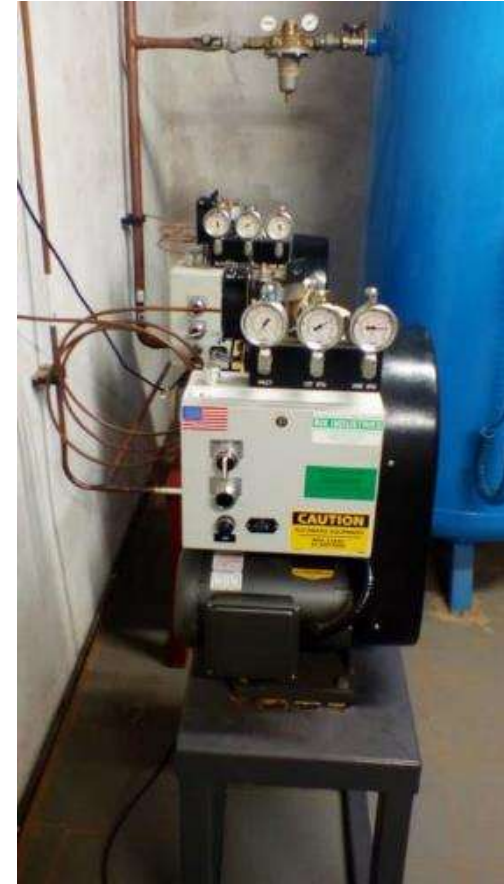
Both boosters are simultaneously operating to fill the cylinders with medical oxygen (94-96% purity)
