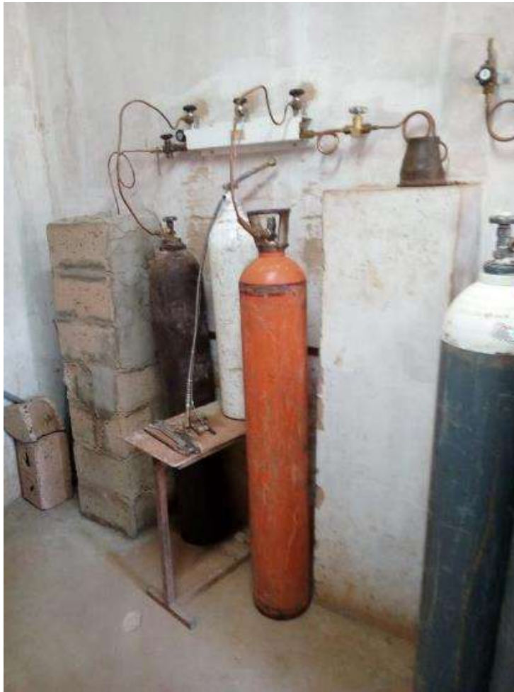
Protective shielding with reinforced concrete of the 2 oxygen loading lines in cylinders for technical staff protection
