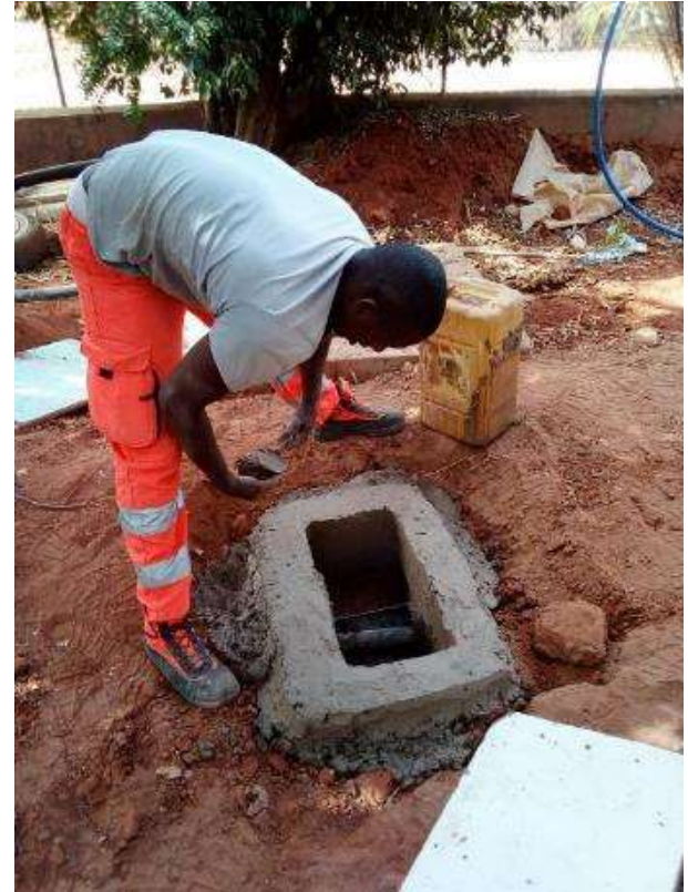
Sewer inspection construction
