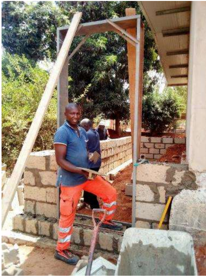
Construction of the cabin containing the general electrical panel for radiology pavilion
